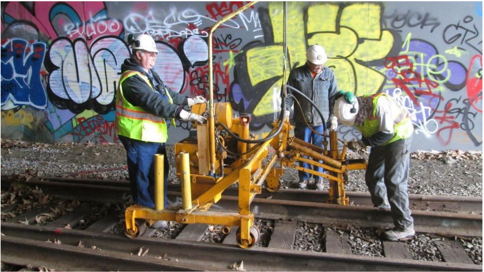
Chris, John, and Matt push ahead pulling spikes with the spike puller despite it slowly dying from a hydraulic leak
