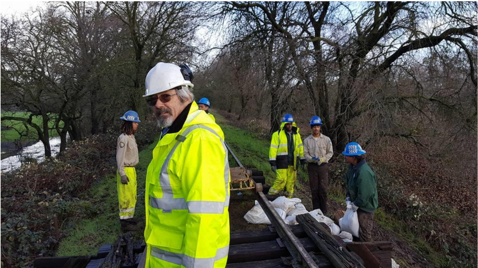
Ed with the CCC crew deploying sandbags
