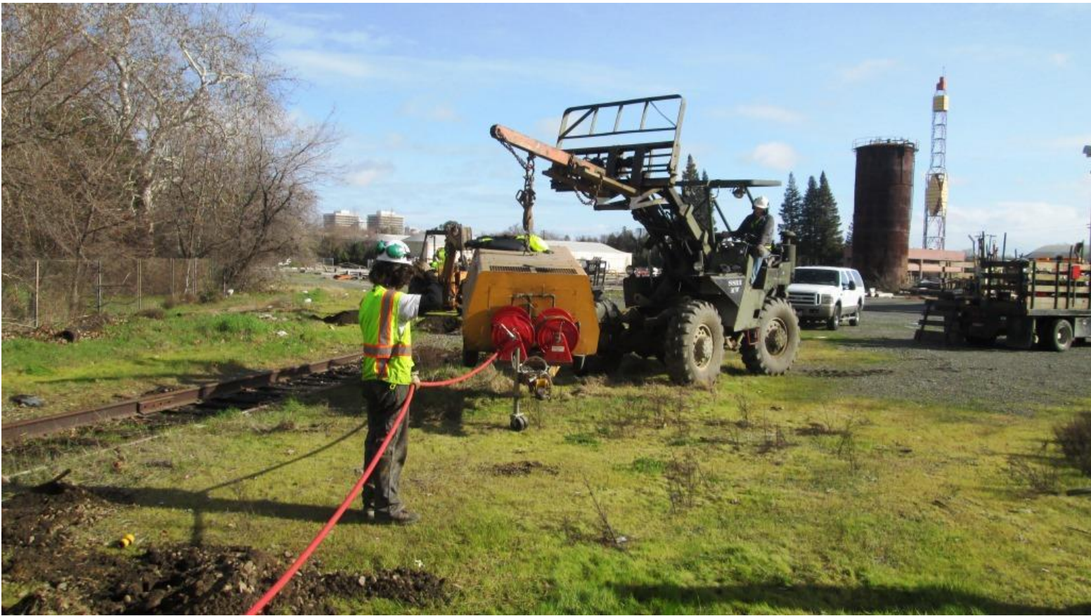
So, Steve grabbed the air-compressor with Big Green and brought it closer as Matt guides the hose – that’s one way to do it...
