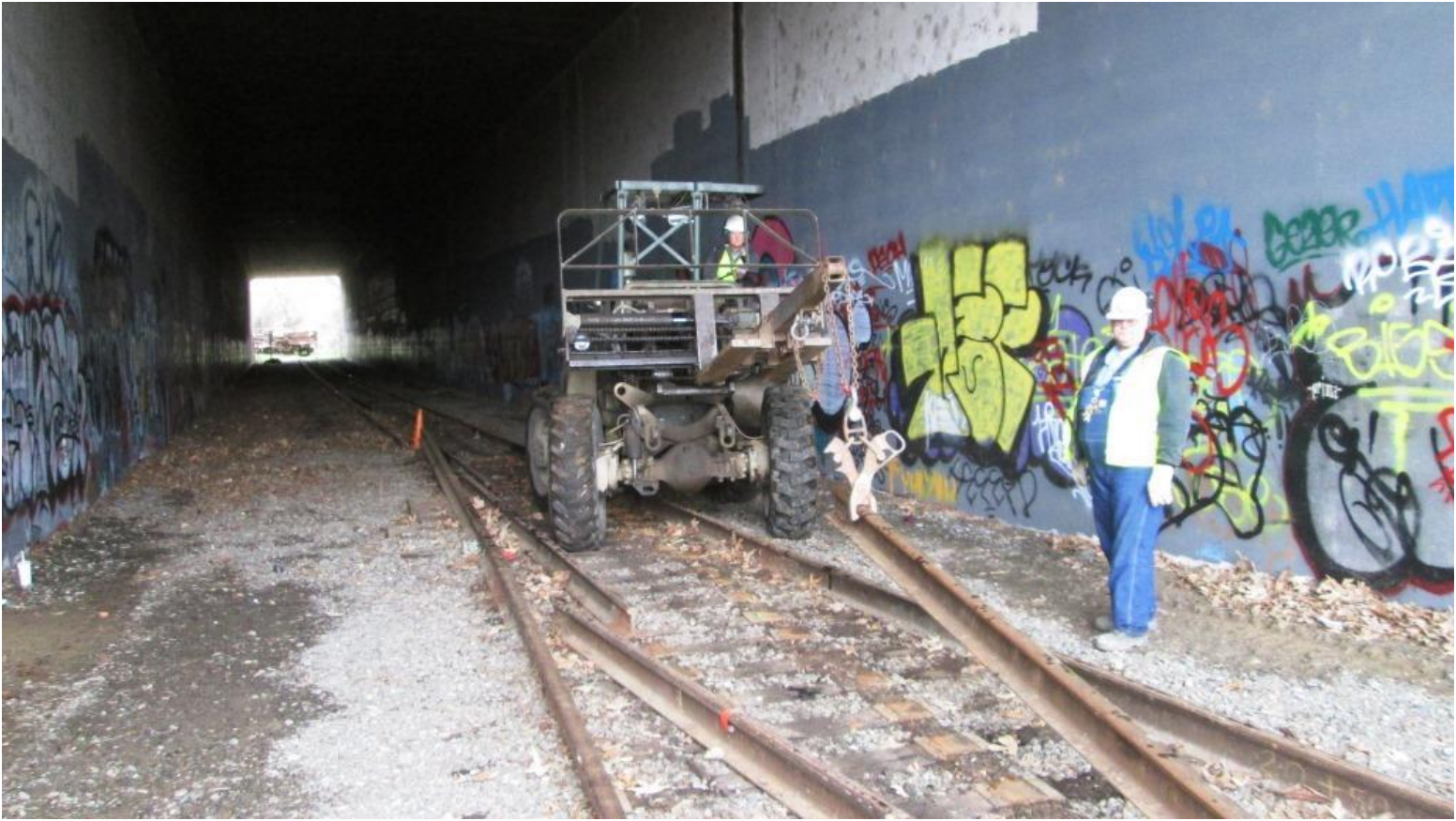
Steve on Big Green starts pulling rails into the tunnel
