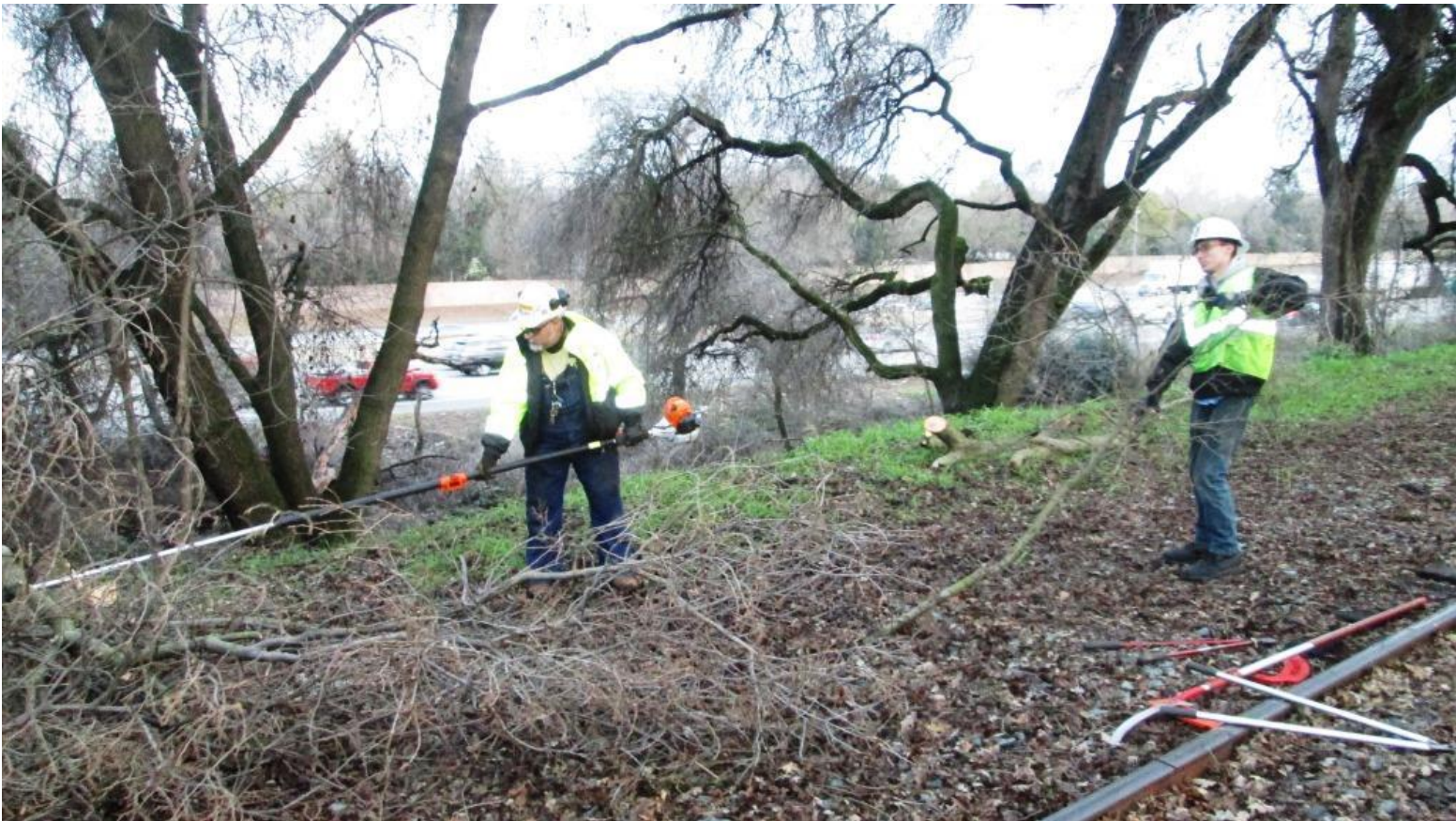
Mike F. and Paul clear away the debris
