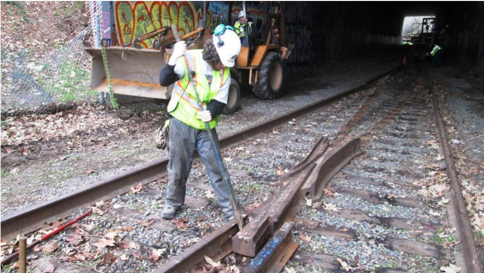
Matt prys the wing-rails off of the frog
