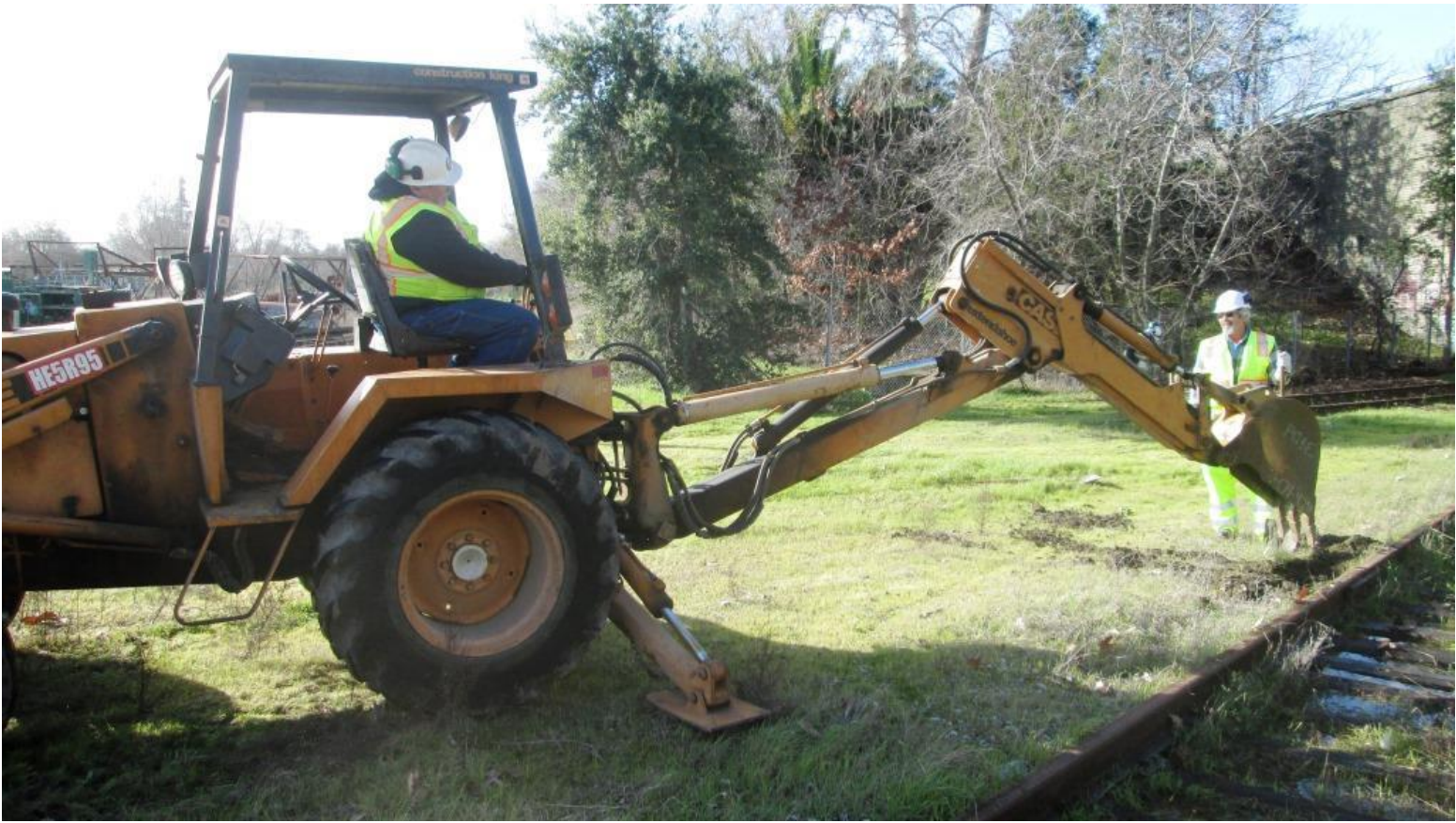
Harry on the back-hoe digs out a rail-joint to make space for the impact wrench to take to remove bolts
