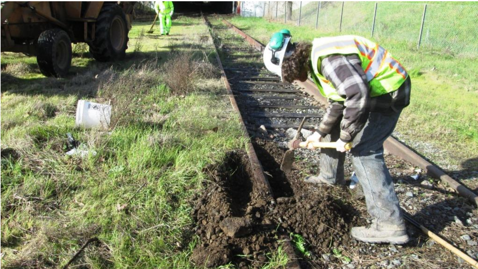
Matt digs out a rail-joint at Setzer
