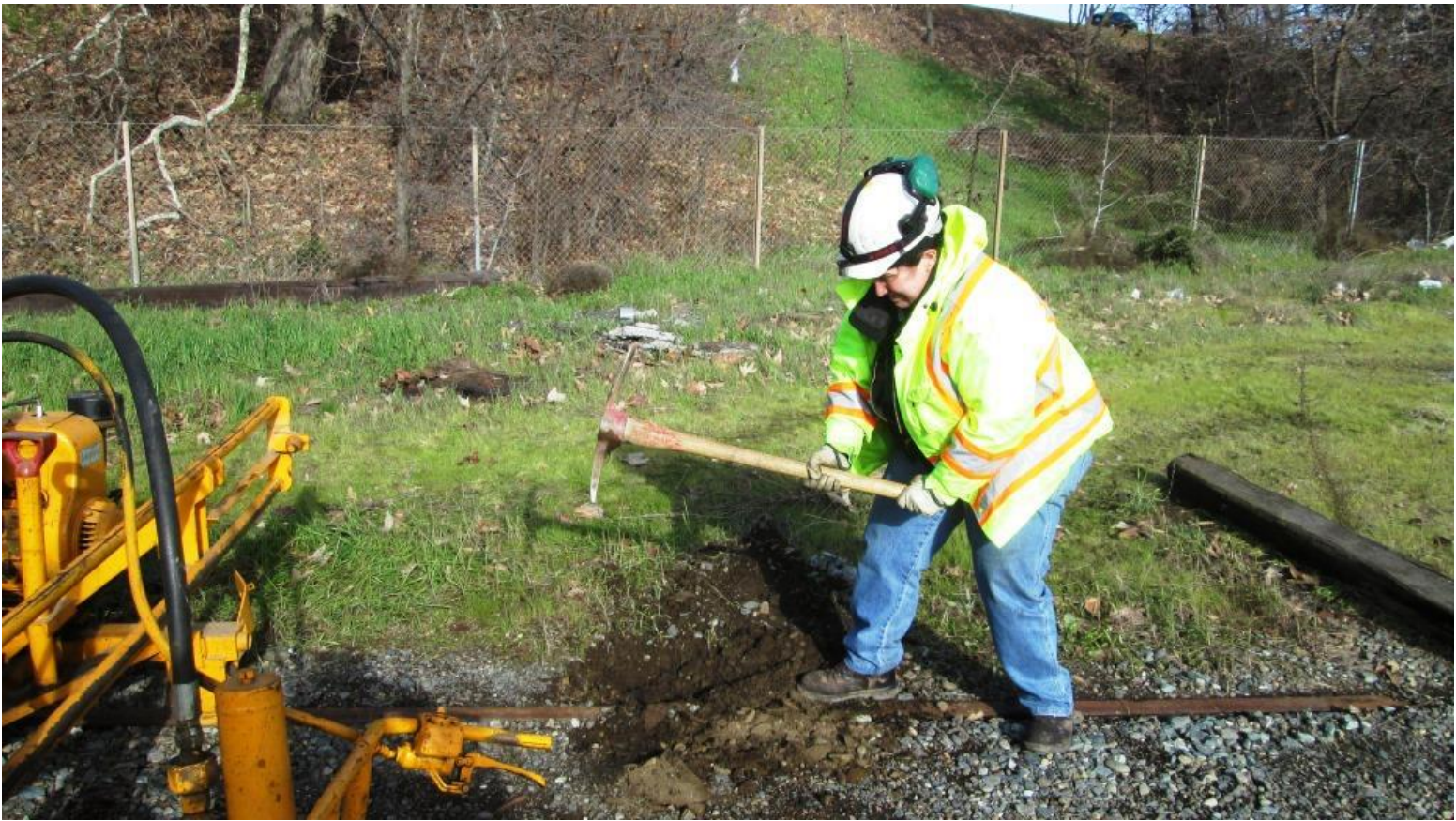
Heather keeps digs out the gauge-side of the rail so that the spike puller can access the spikes
