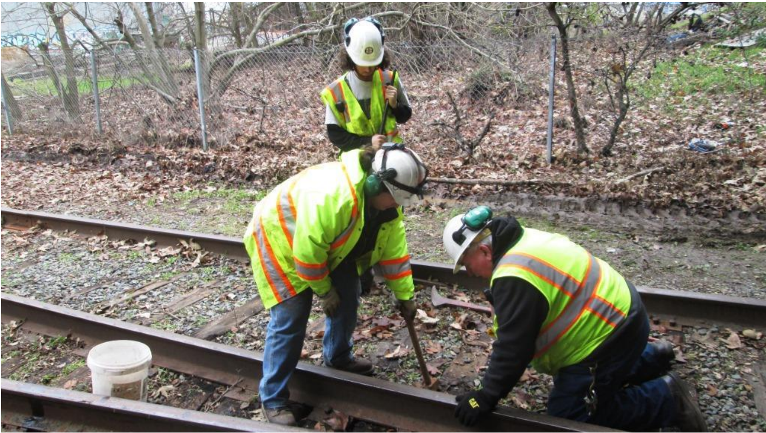
Heather and Harry fight with a particularly stubborn spike along the rail leading into the frog
