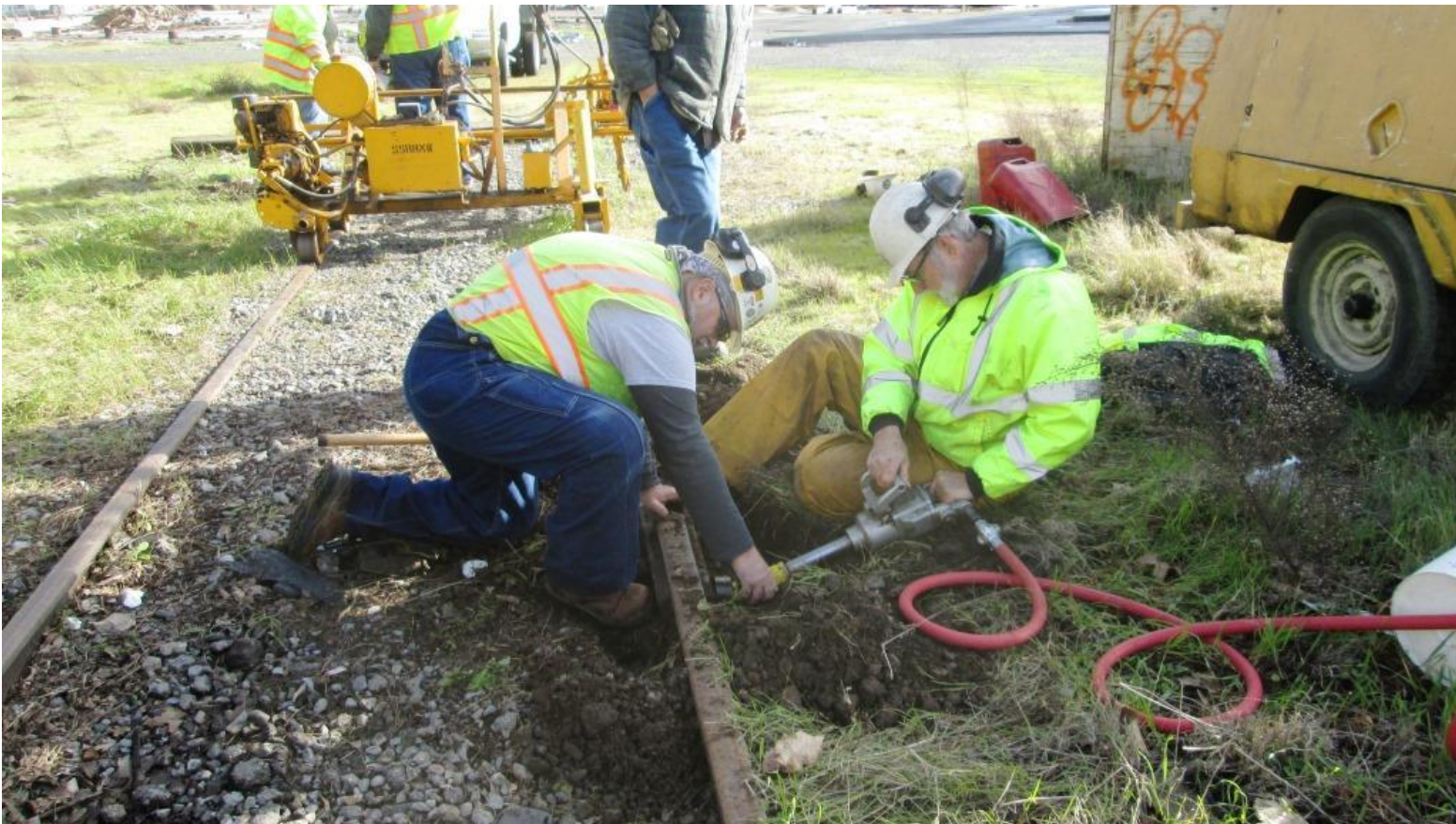
Mike F. and Alan use the pneumatic impact wrench to remove the bolts
