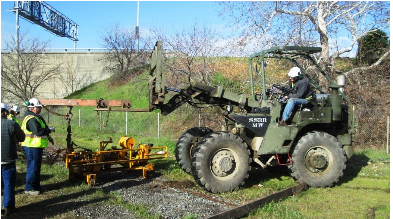
Steve on Big Green retrieves the spike-puller from the truck and sets it on the rails
