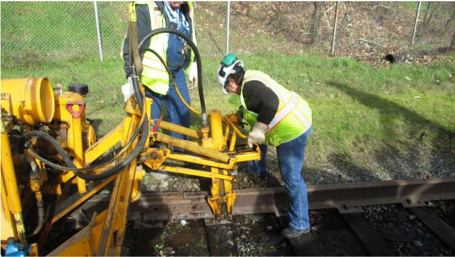
Pam uses the spike puller to pull spikes
