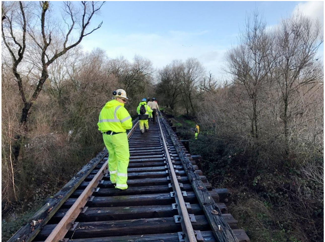
Mike F. with the CCC Crew on the trestle near the spot of the levy leak
