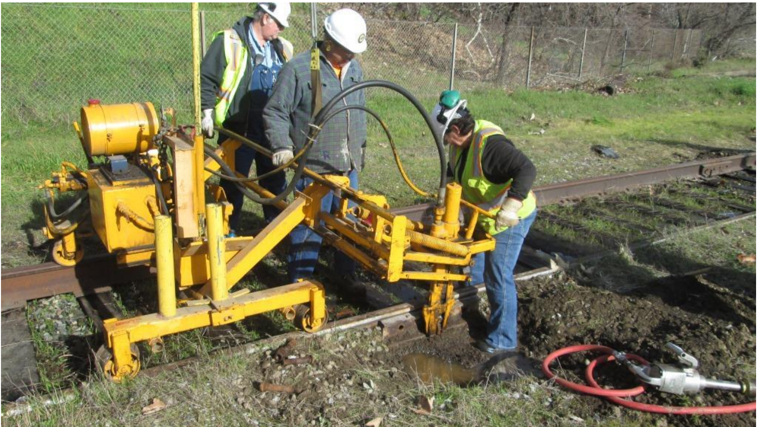
Pam races down the track pulling spikes at a record pace
