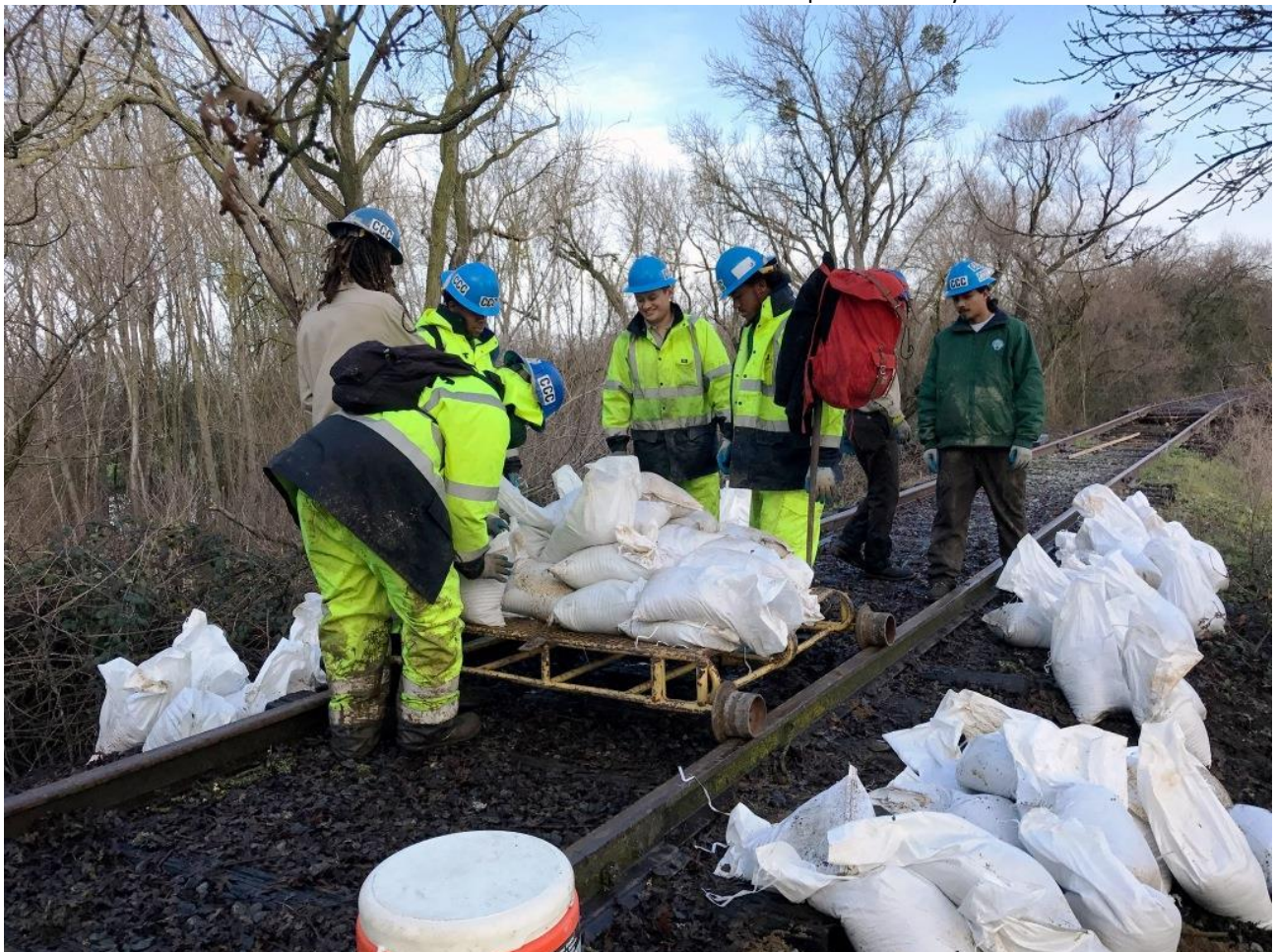
The CCC Crew unloading sandbags off the Nolan track-cart
