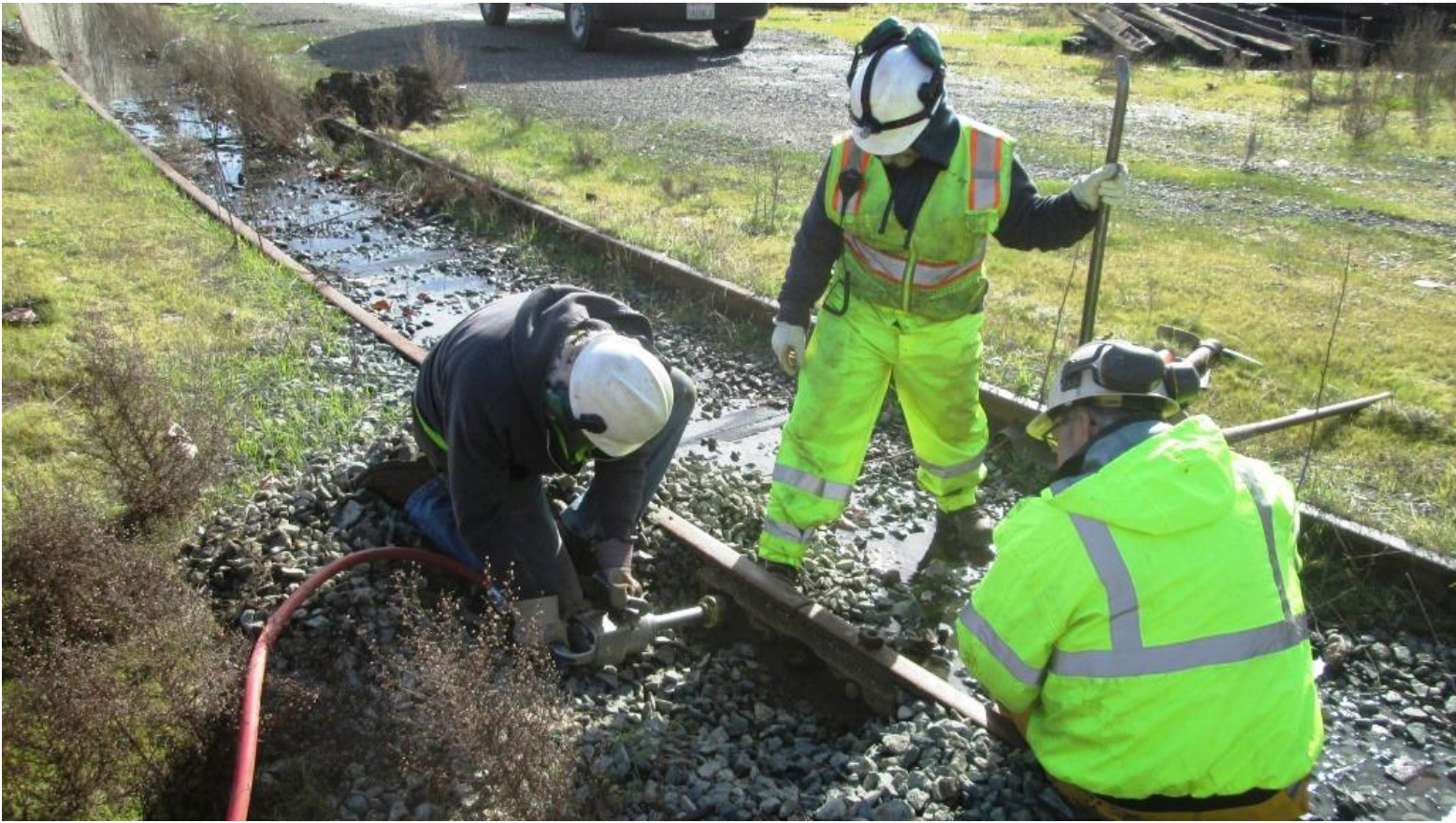
Joe holds the bolt-head with his foot as Steve unwinds the nut
