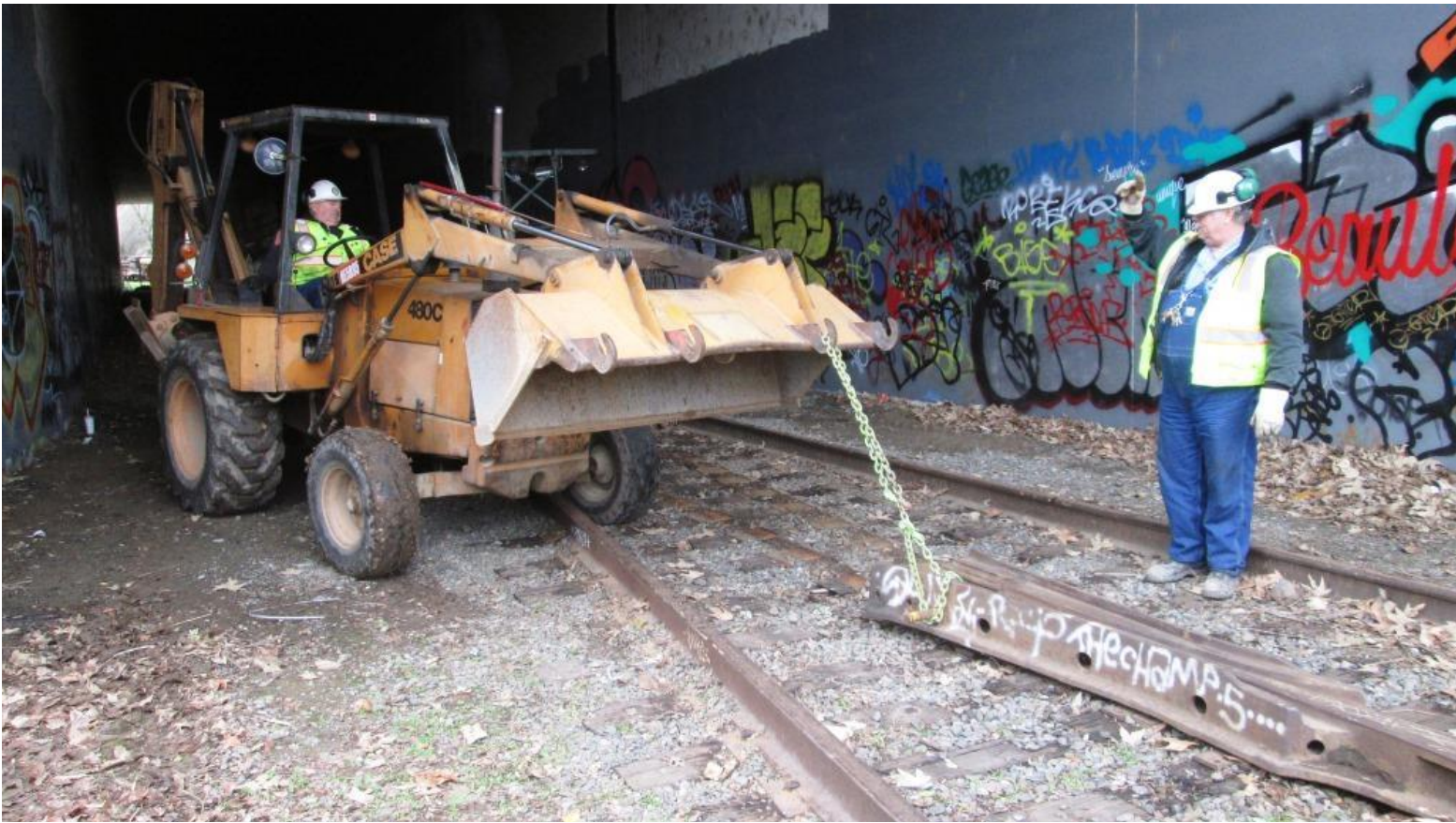
Harry on the back-hoe pulls the frog into the tunnel
