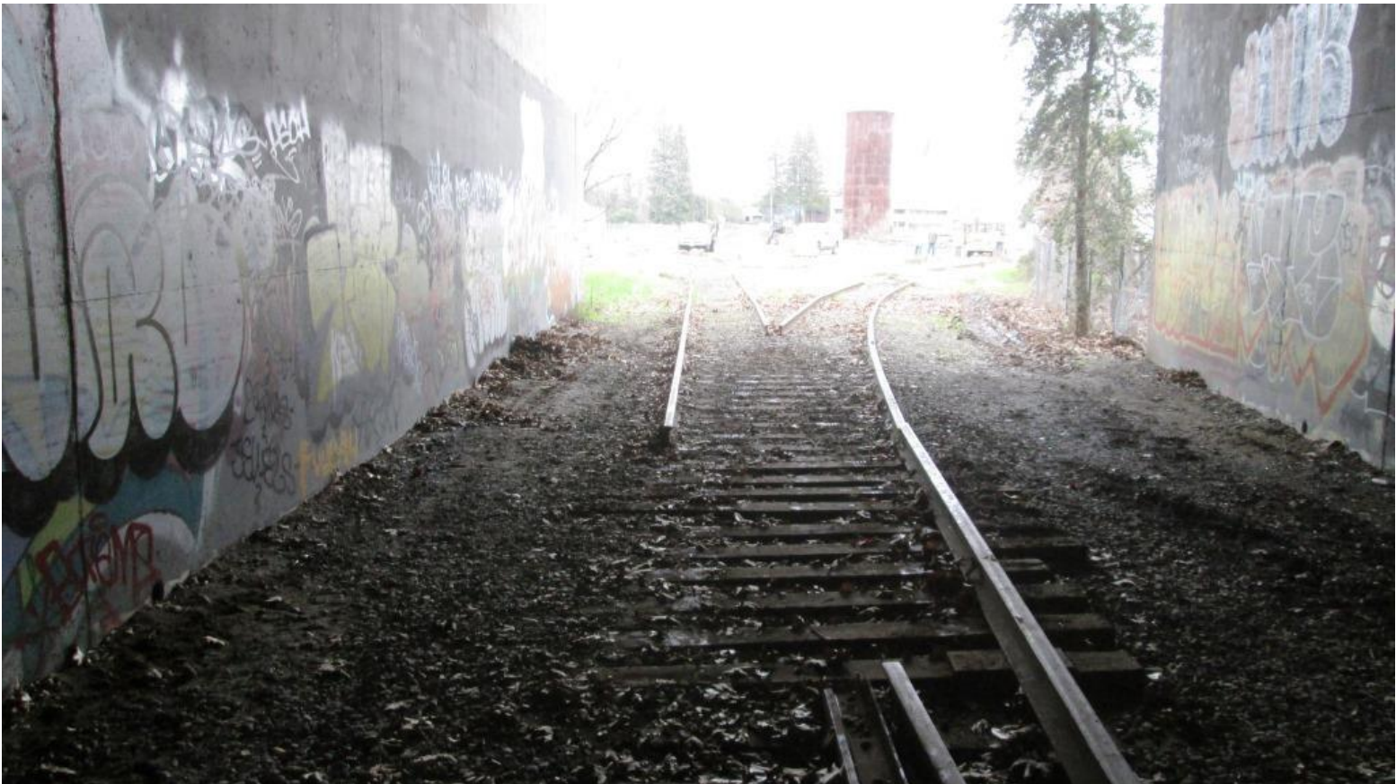
There's not much left of the switch...
