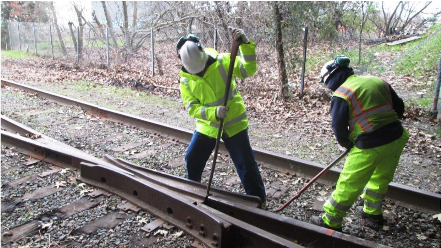
Ed and Joe pry the un-spiked rails out from the frog
