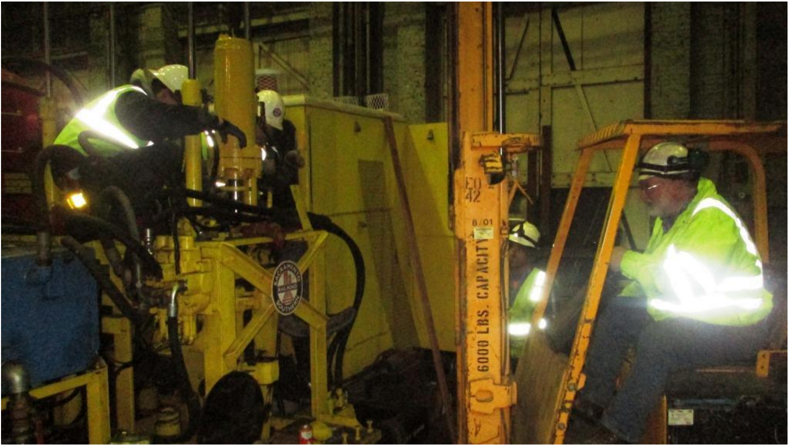
Paul and Matt on top of the shear guide the cylinder into place which is suspended by the forklift under Frank's skillful touch
