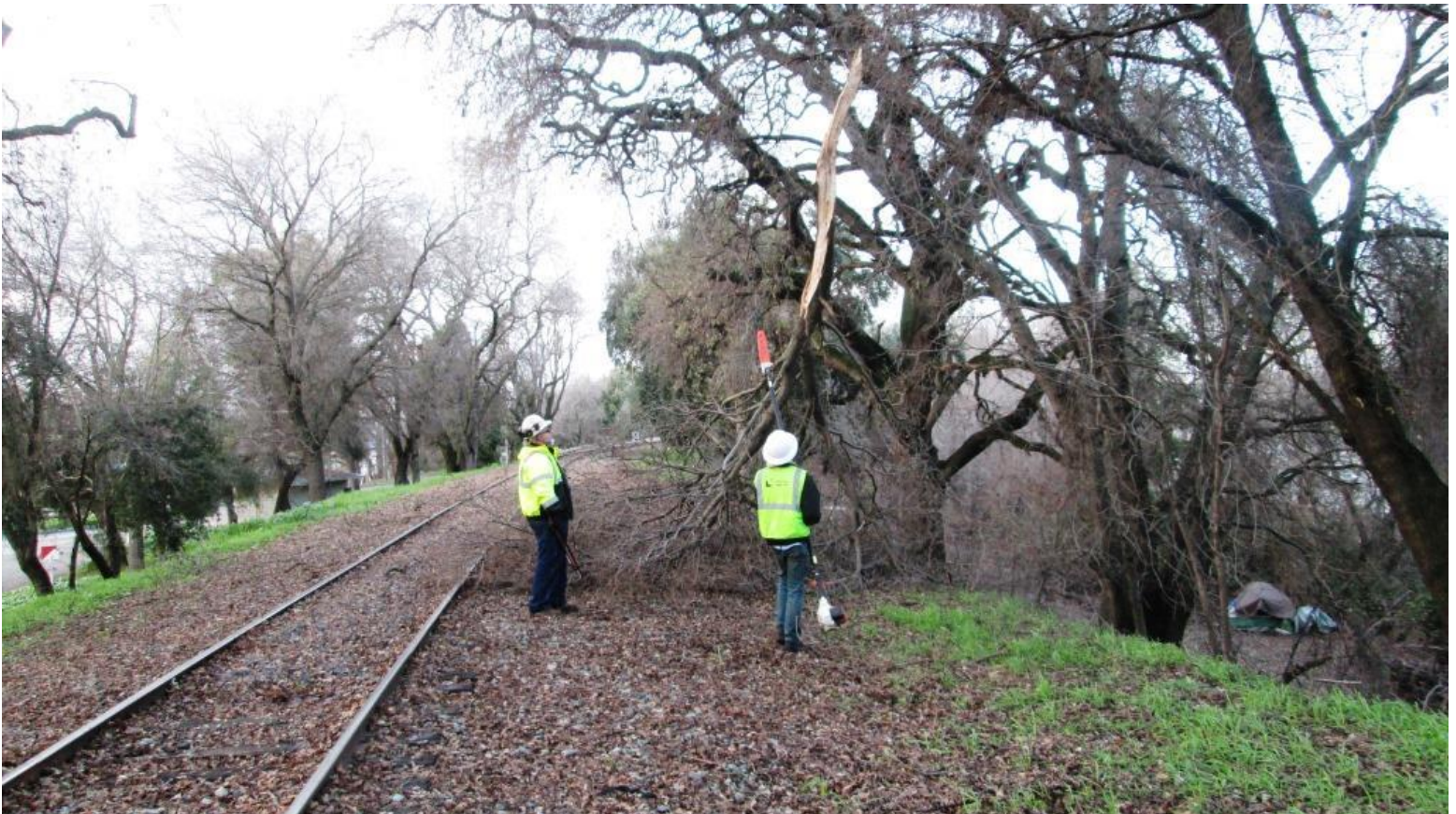
Meanwhile, up on the SSRR Mainline, Mike F. and Paul prepare to remove a broken branch fouling the line
