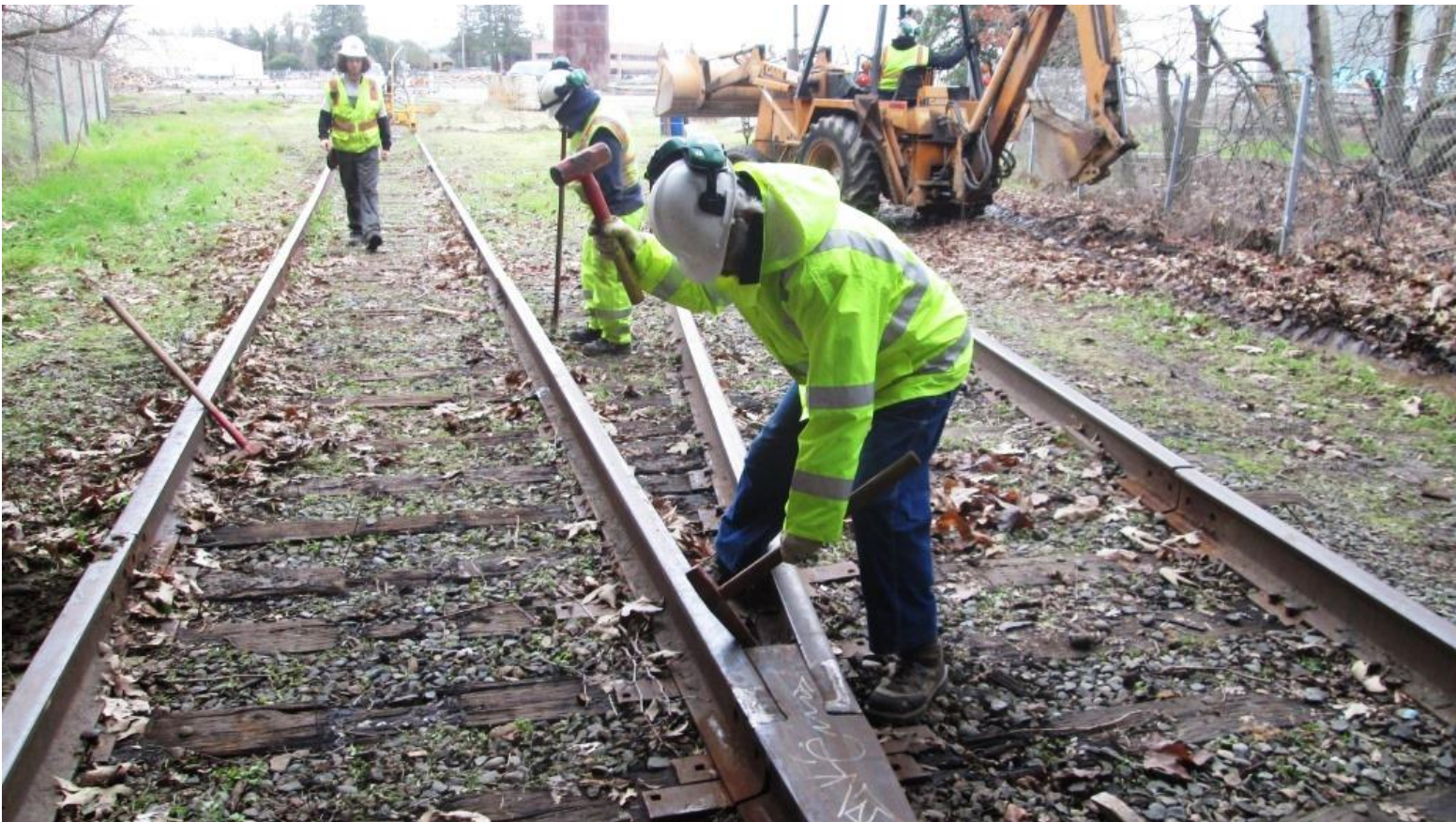
Ed uses a track-chisel to break an old bond-wire welded between the frog and rail
